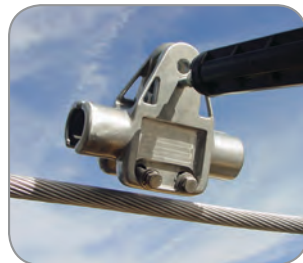
3. With the HIBUS Suspension in the open position, locate the unit on the conductor
