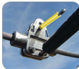
7. Tighten the captive bolts on the HIBUS Suspension to the specified torque
