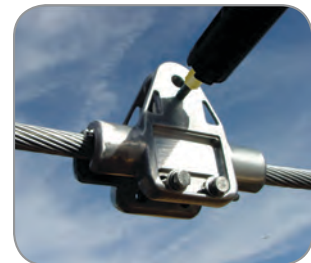
4. Once in position, rotate the "Hot Stick" (with Live-line Attachment Tool attached) in a clockwise direction until the HIBUS Suspension is fully closed
