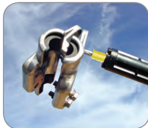
2. Secure the HIBUS Suspension to the "Hot Stick" using the Live-line Attachment Tool
